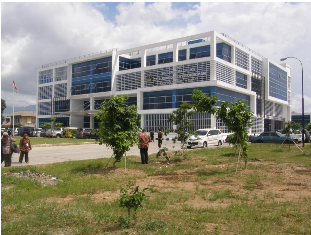
Photo 10 The base isolated Public Works Agency office of Sumatera Barat. Photo: Phil Glassey, GNS.
