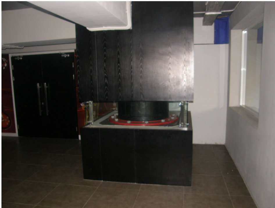
Photo 7 A rubber base isolator on display in the basement of the Ibis Hotel. Photo: Phil Glassey, GNS.
