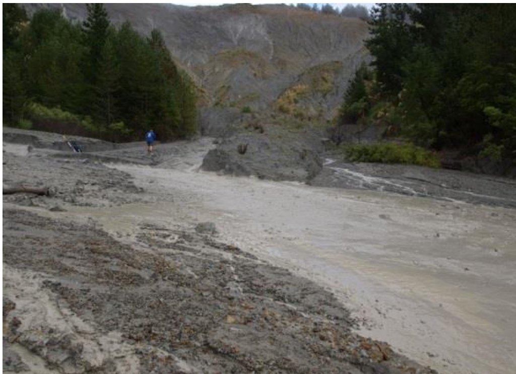
Figure 8 Fresh failures on headwall scarp (top of photo) resulting in a debris flow and infilling of the channel floor during a prolonged period of heavy rainfall.
