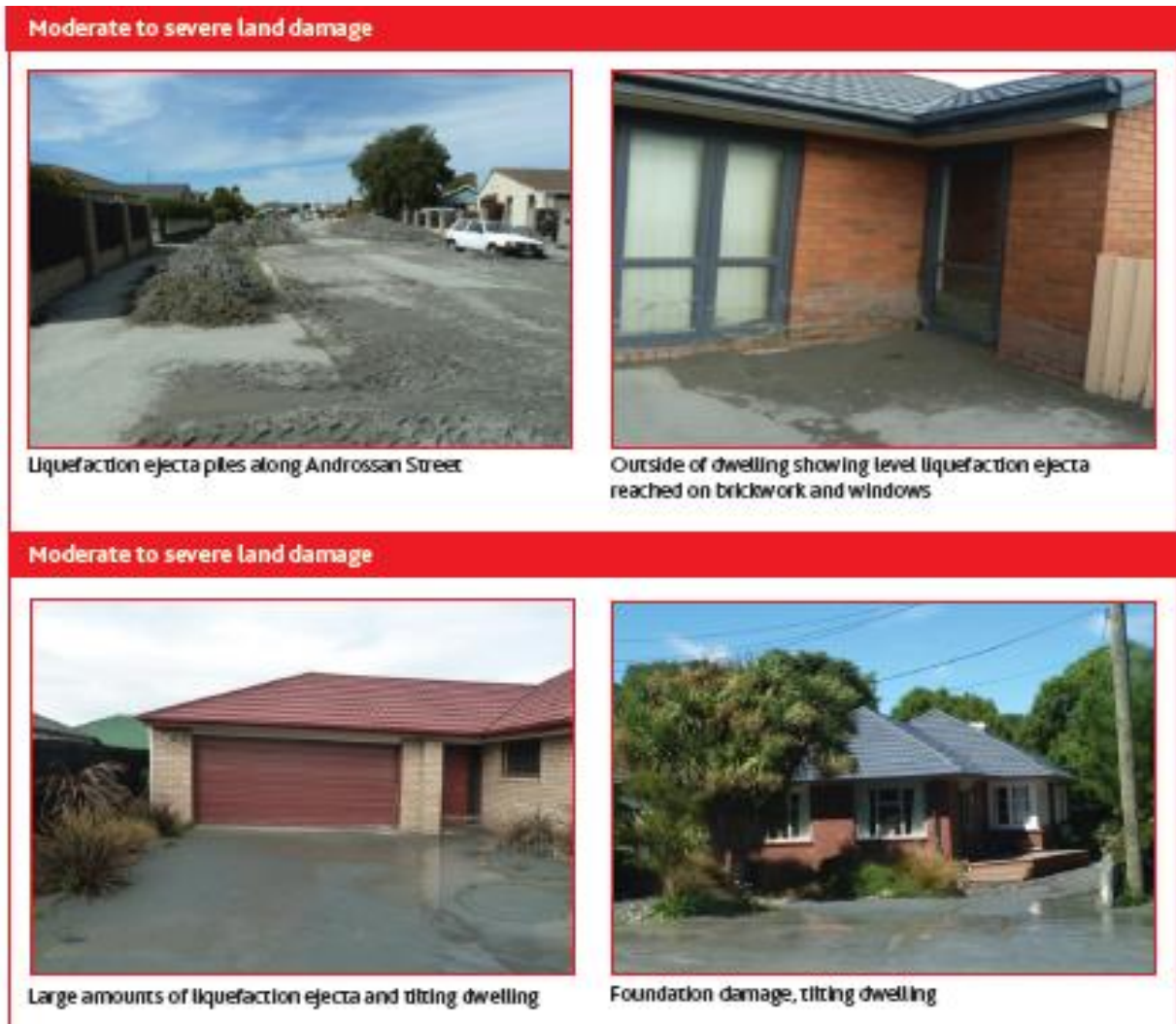
Figure 8 Examples of moderate to severe land damage (LSN >30) in Christchurch following the M6.3 February 22, 2011 earthquake.
