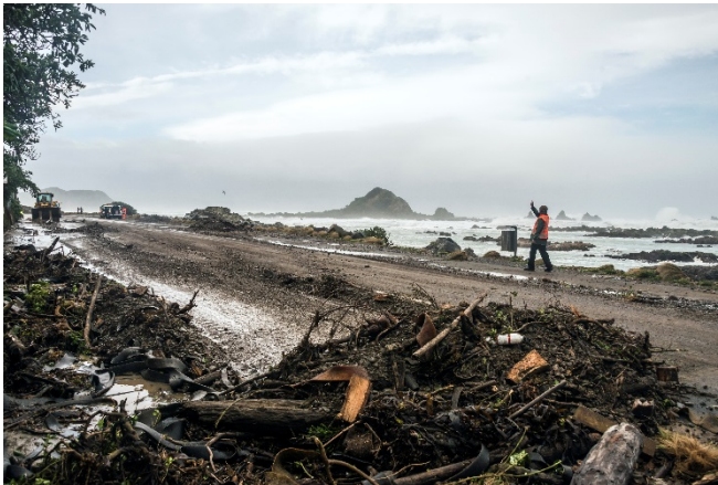
Island Bay storm damage June 2013. Source NIWA.
