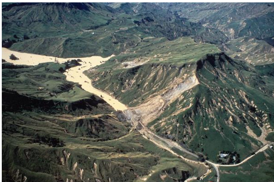
Figure 6 Waerengaokuri Valley after Cyclone Bola (March 1988). A large landslide blocked the valley outlet, forming a lake that flooded the valley which required draining by mechanical removal of the landslide debris
