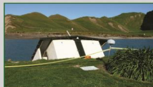
Figure 8. Half of the Kairikau Beach Camping Ground was washed away.
