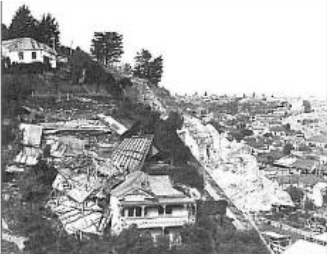
Figures 1 – 3 Examples of landslides from Bluff Hill triggered by the 1931 Napier earthquake:
