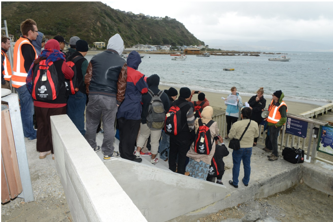
Figure 4 Damage to Island Bay sea wall and the community response being explained by Nicci Wood (WCC) and Kate Crowley (NIWA).
