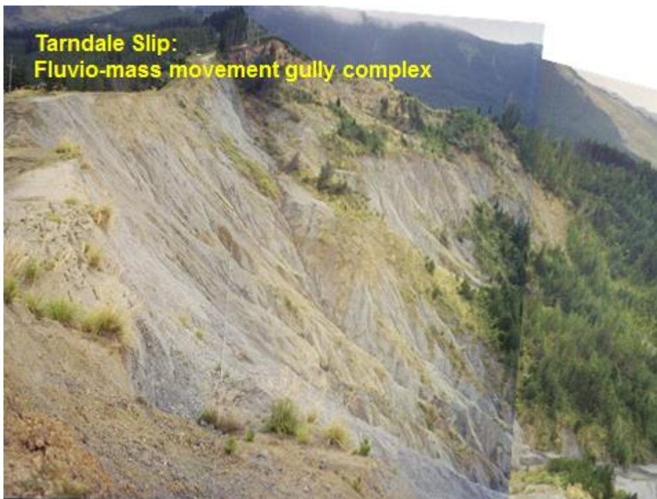
Figure 5 Large scale rotational slump failure of a section of the headwall.
