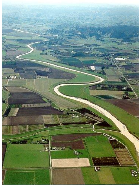
Figure 1 The Waipaoa River Flood Control Scheme near Patutahi
