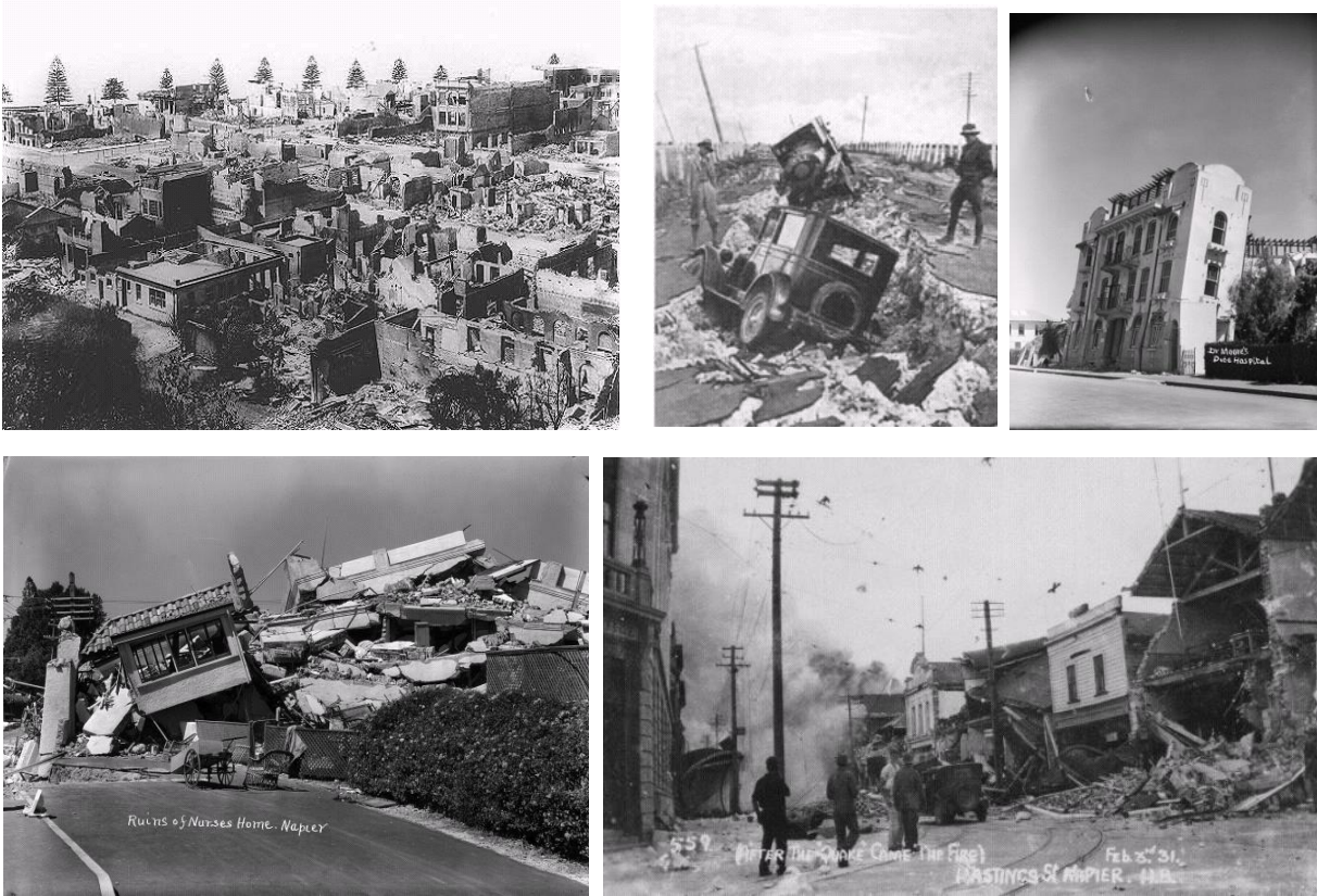
Figure 1 Damage in Napier city following the 1931 earthquake. From Alexander Turnbull Library collection http://www.natlib.govt.nz/collections/highlighted-items/hawkes-bay-earthquake-1931
