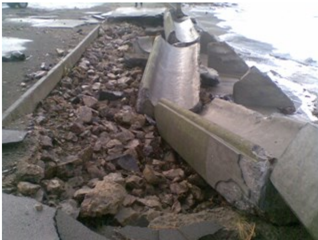
Some of the storm damage to the Island Bay seawall (Source WCC).
