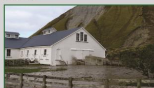
Figure 9. Damage to Aramoana Woolshed. Photo courtesy of CHBDC.
