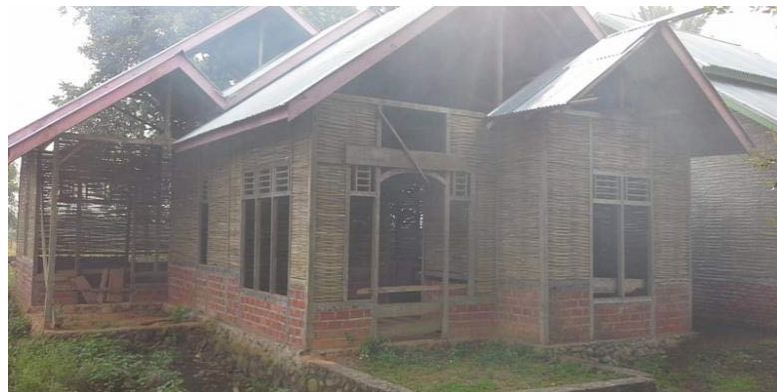
Figure 2.20 Rumah bidai (bamboo house) under construction (photo credit: Ade Wahyuni)
