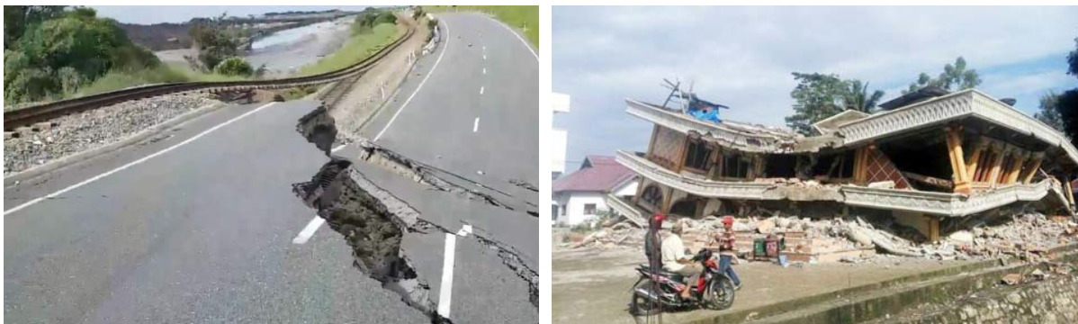
Figure 2.6 Damage to road and rail infrastructure, Kaikoura earthquake (left) and collapsed 3-storey building following the Pidie Jaya earthquake (right). (photo credits: Kelvin Berryman (L), Iman Satyarno (R))
