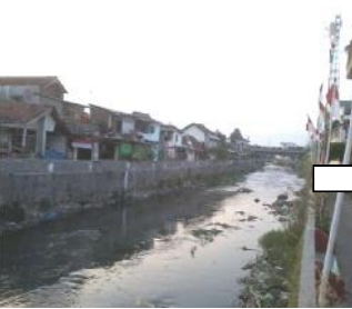
River needs restoration
