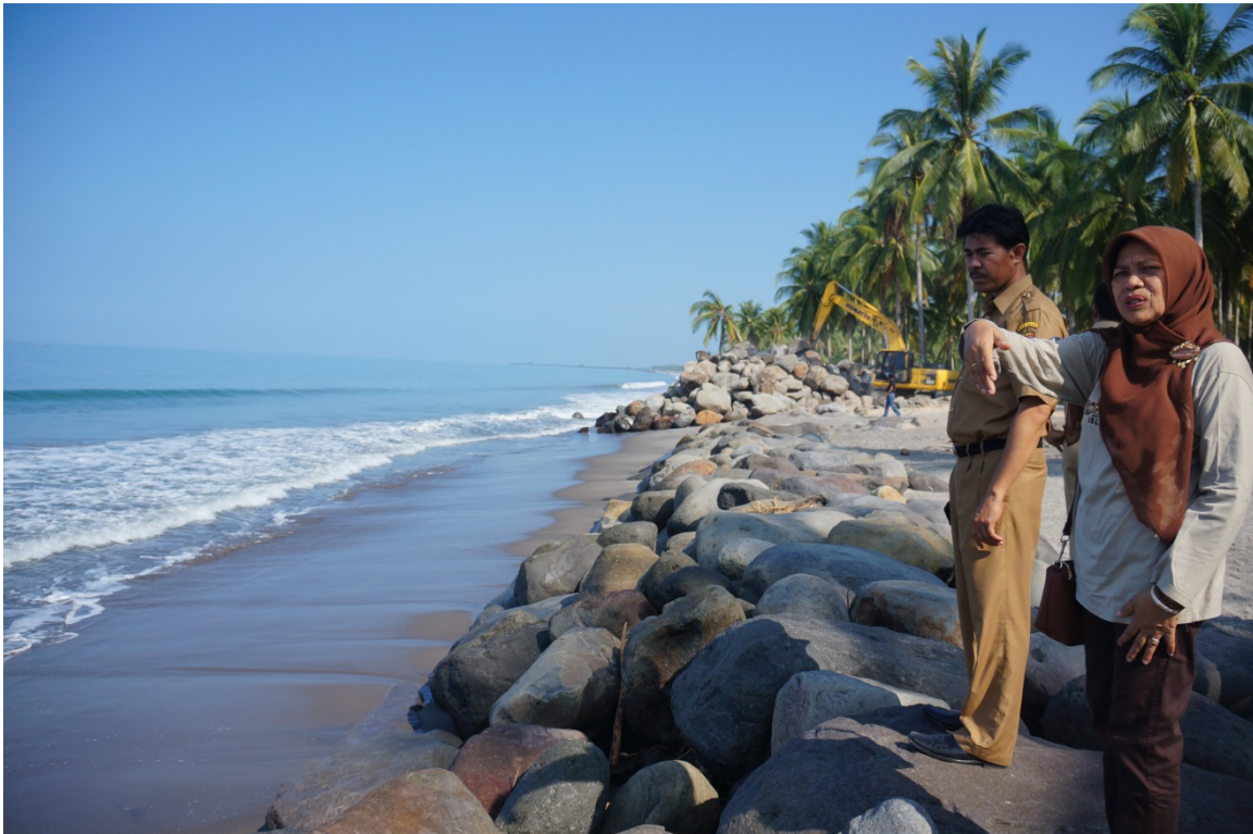
Rockwork structures being built, North Tiku Beach (photo G Maylda Pratama)
