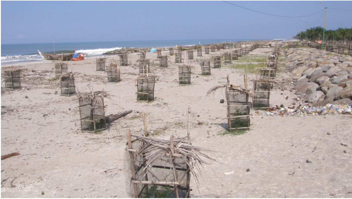
Erosion remediation of tree planting and rock structures is being adopted at North Tiku Beach. Up to 105 households agreed to be relocated from this location due to erosion.
