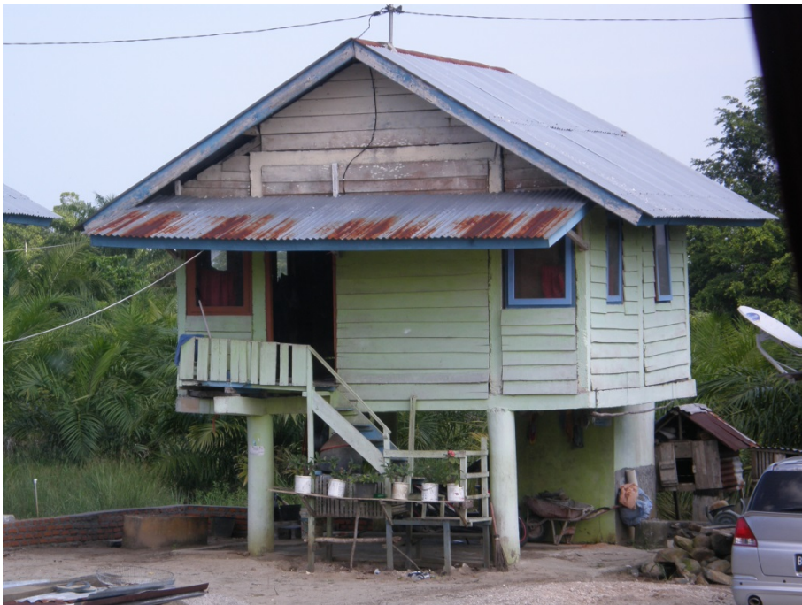
The re-located households were moved inland from North Tiku Beach to a flood prone area and have floor levels elevated above the potential flood levels.
